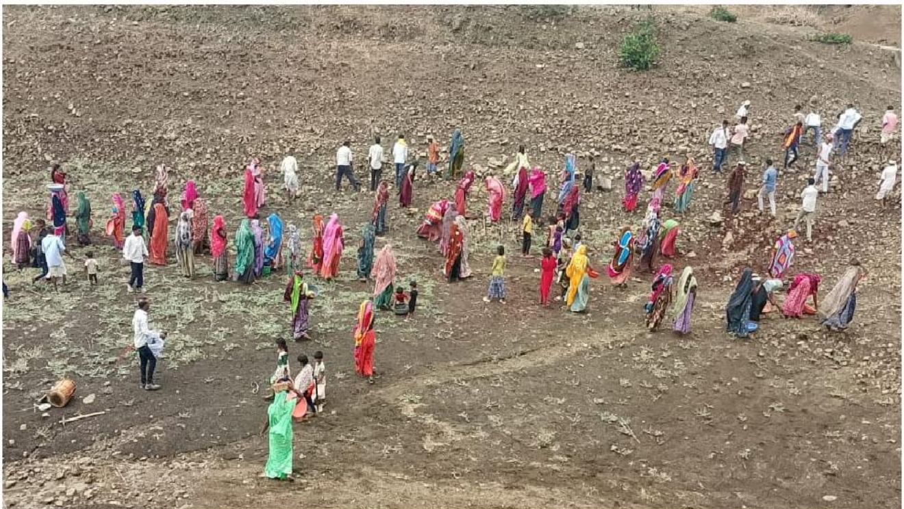
Guided by the indigenous tradition of Halma, community members joined hands in voluntary labour to construct water saving structures
